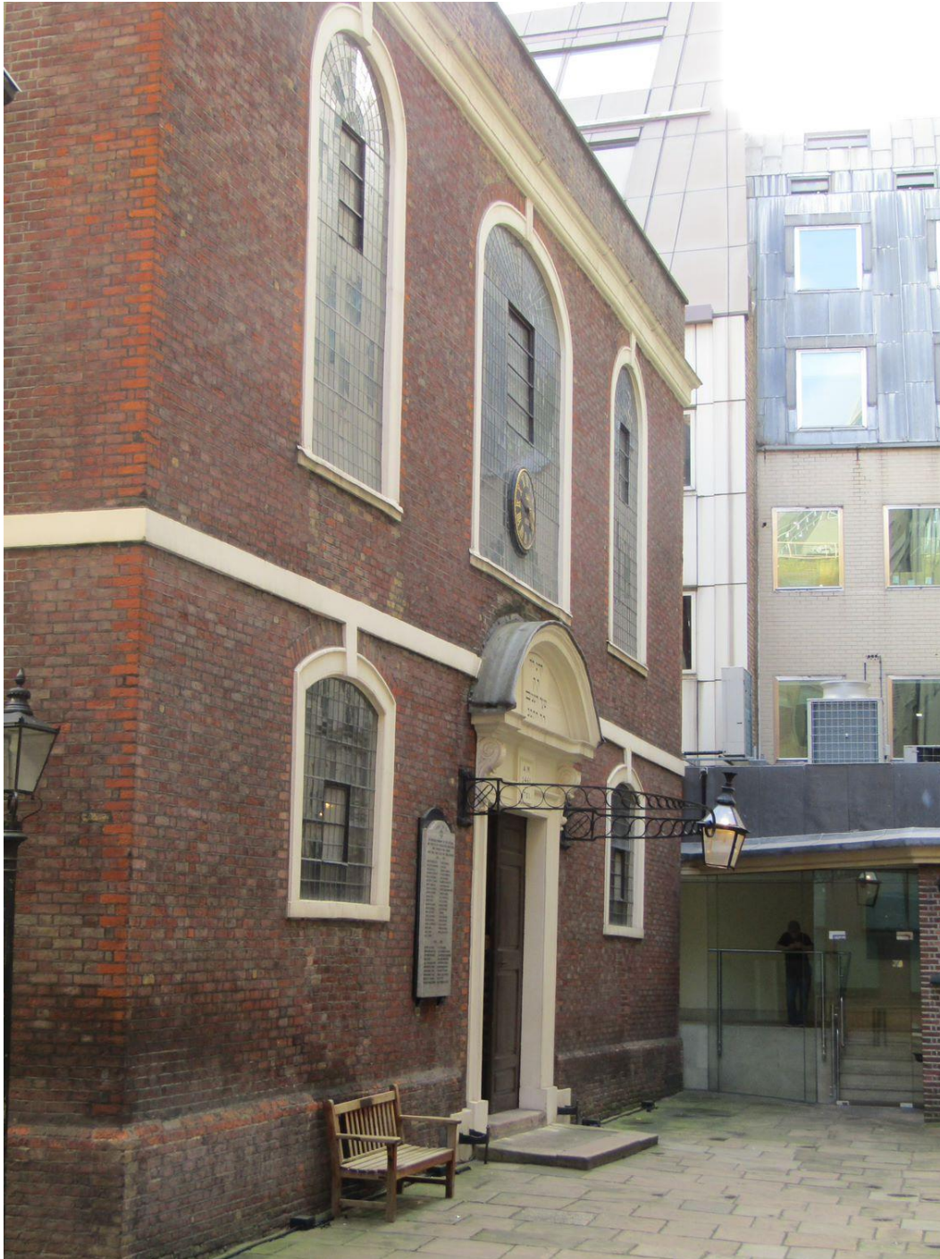
Figure 7: Bevis Marks Synagogue, western elevation
